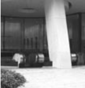
Outside escalators at 9 West 57th Street, meant for planned LDS Church use.
